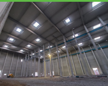
Indoor of the containerboard warehouse
