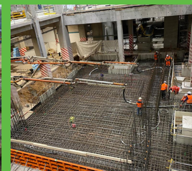
Foundations for the winder
