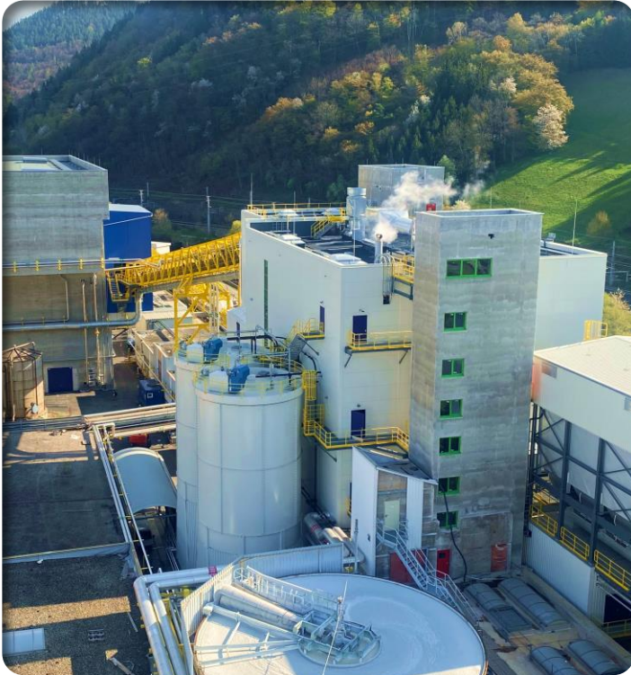
Bruck waste-to-energy facility
