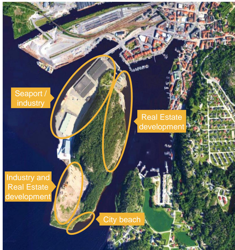
Overview of Sauøya 0.71 km 2 , Halden city, Norway
