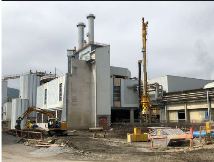
Waste to energy plant being installed in Bruck, Austria
